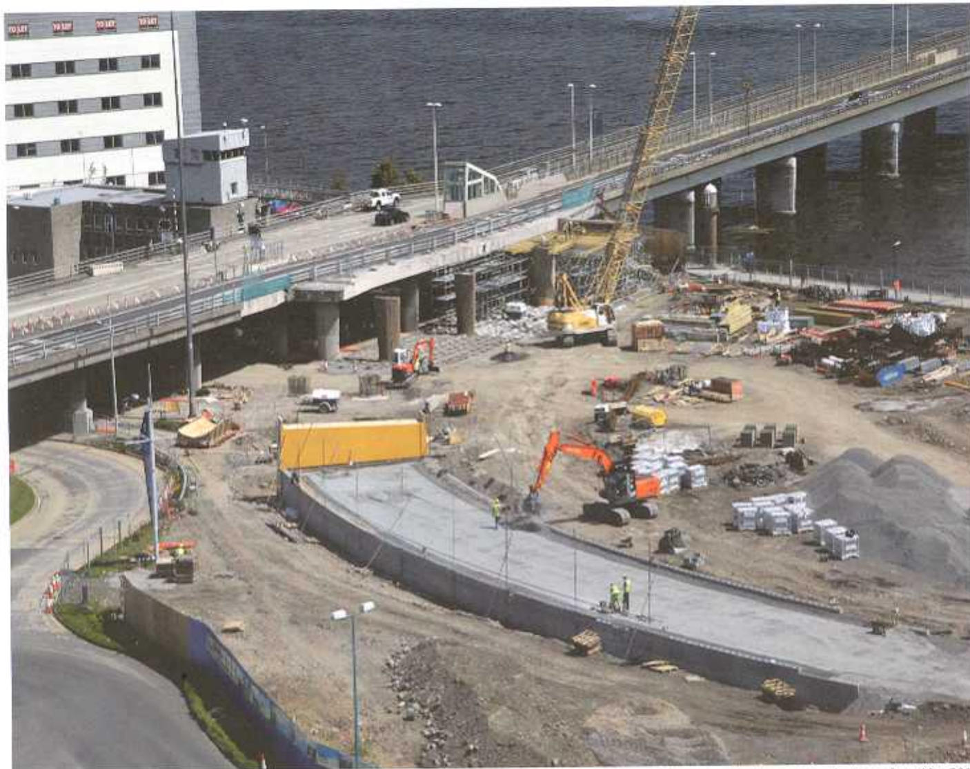
Construction of the new West bound off ramp - Dundee Waterfront May 2011
