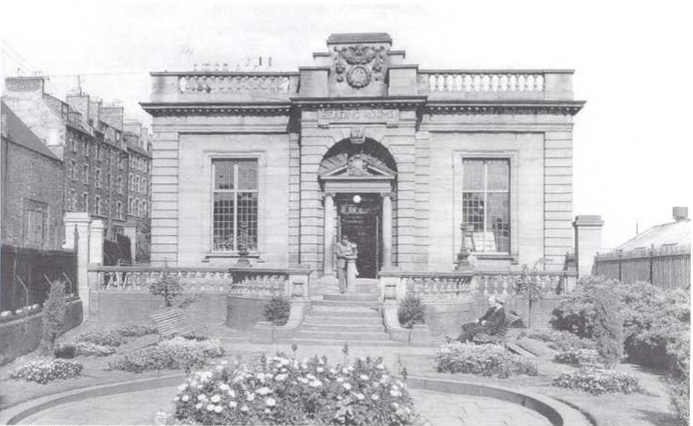
St Roques Public Library, Blackscroft Circa 1950 - © DC Thomson
