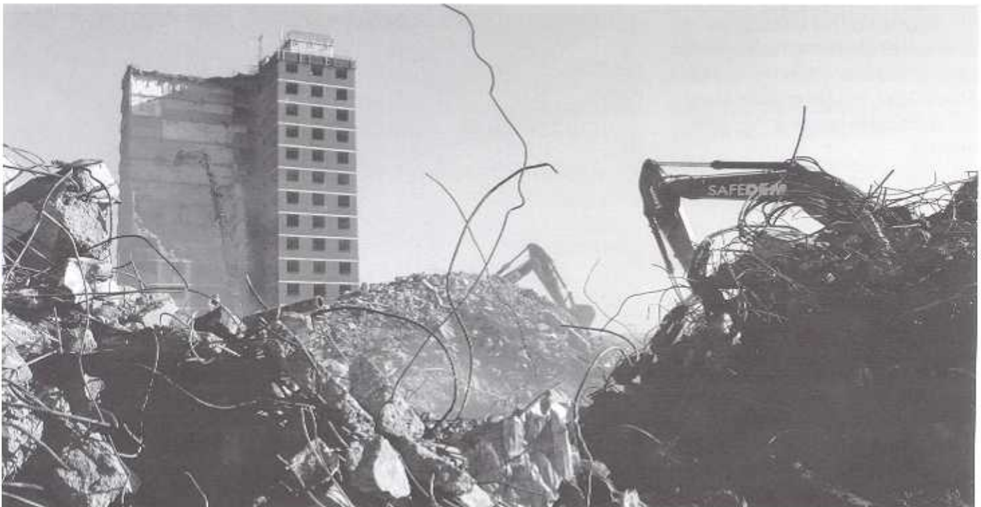
Hillside Court during demolition
