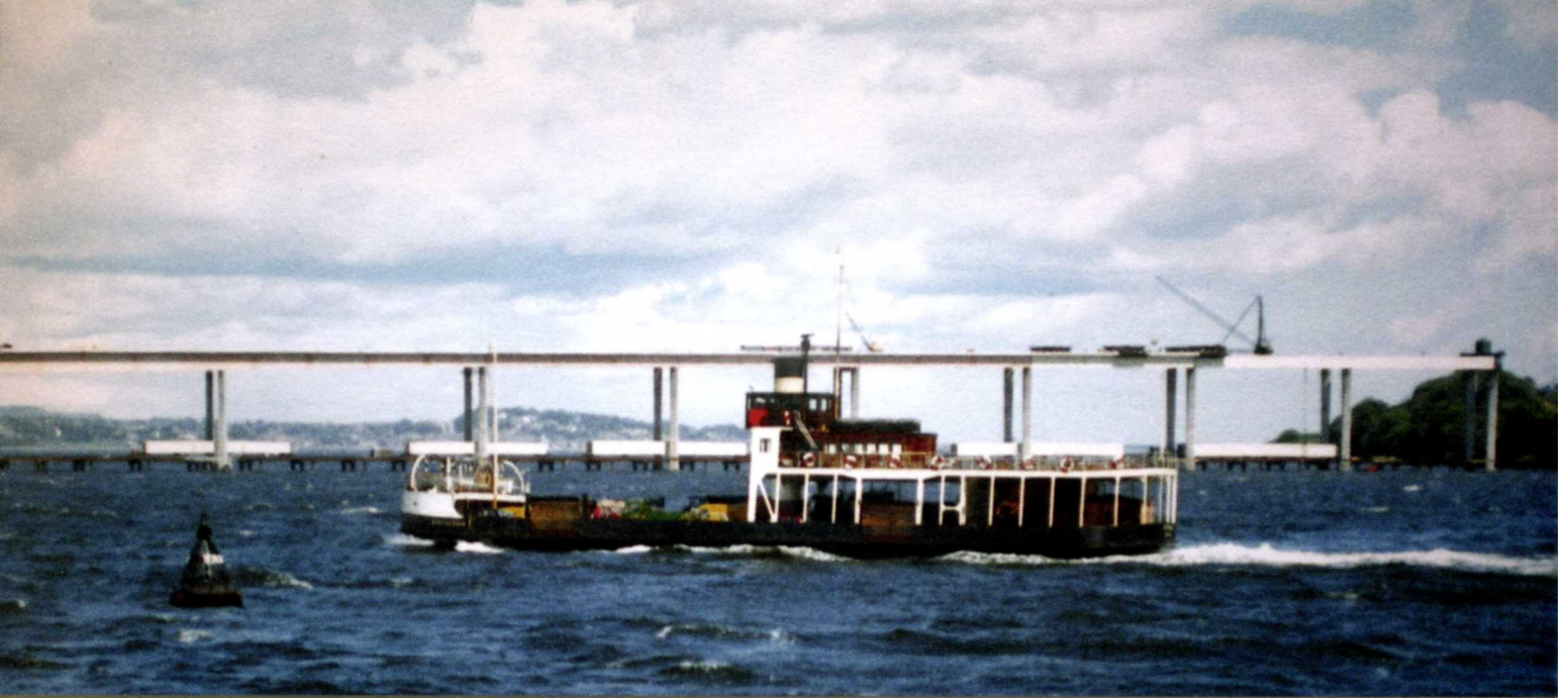
▲ Tay Road Bridge under construction and MV Scotsraig. Photo: Bob Kennedy
