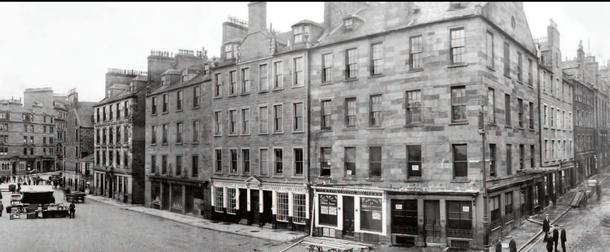
▲ A horse drawn cart can be seen passing the original D P & L building in Shore Terrace. Photograph taken circa 1914.
