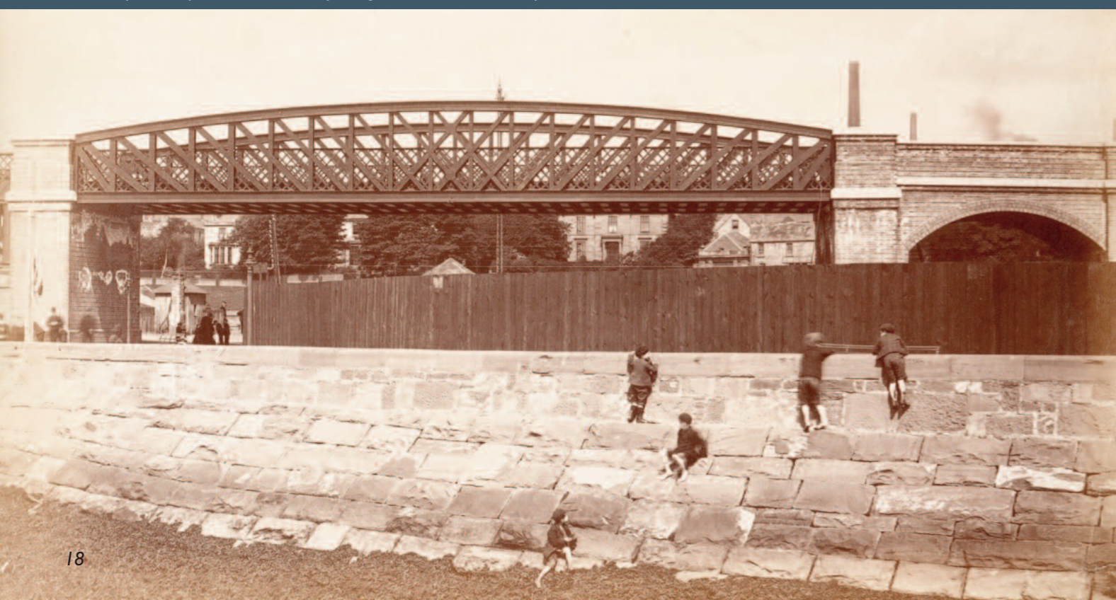
Esplanade span of the second Tay Bridge, since altered. Courtesy of Network Rail
