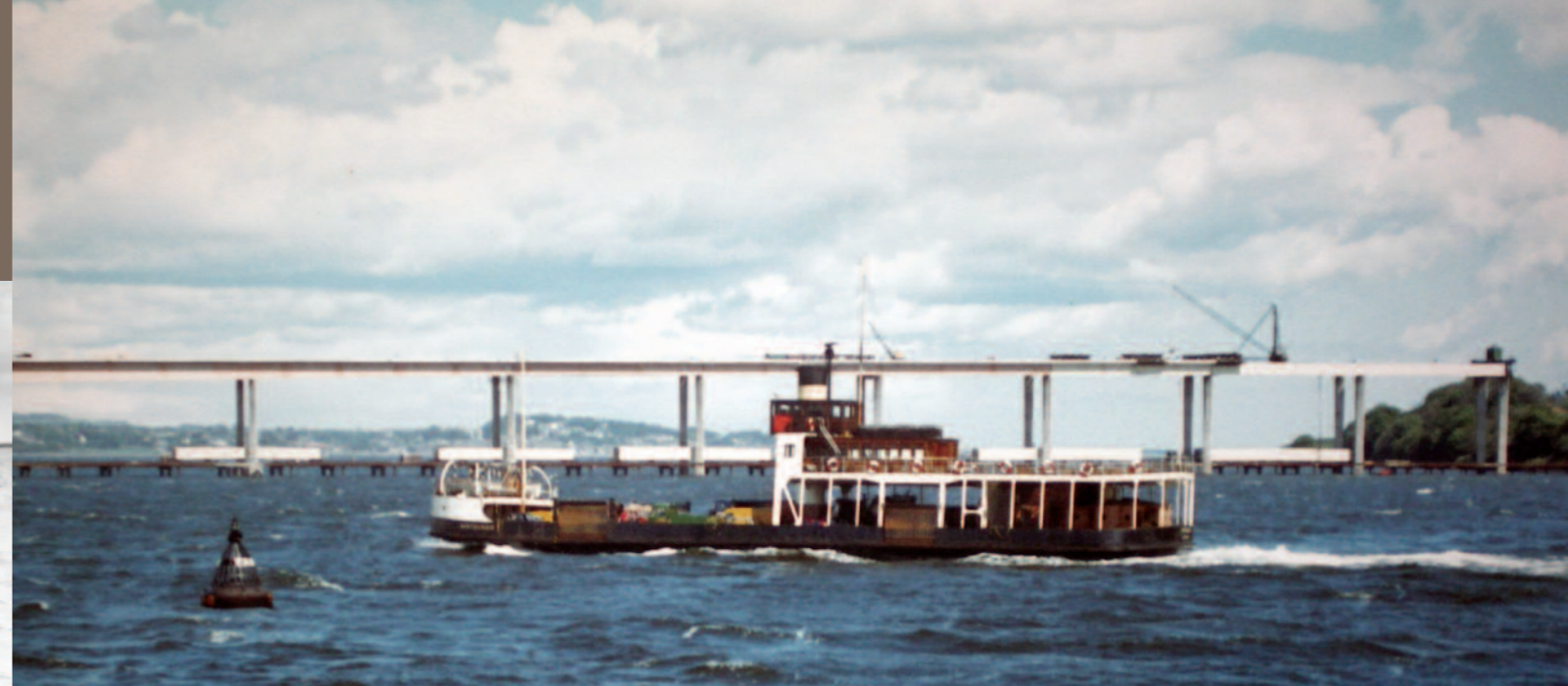
Tay Road Bridge under construction and MV Scotsraig . Photo: Bob Kennedy
