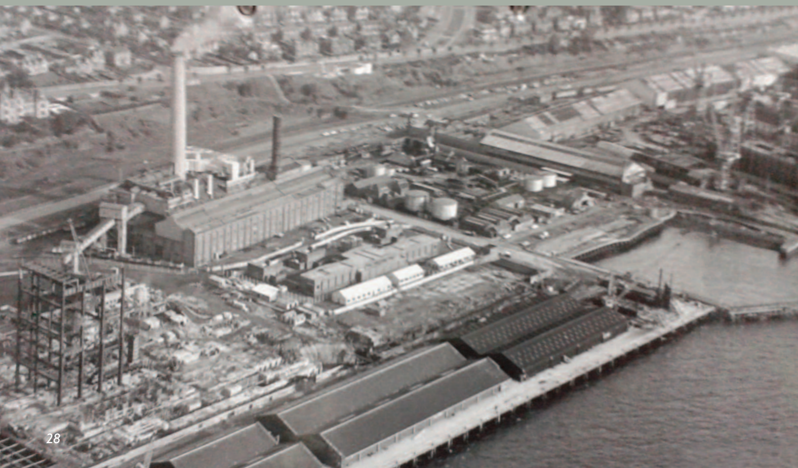
▼ Carolina Port A showing Carolina B under construction circa 1963
