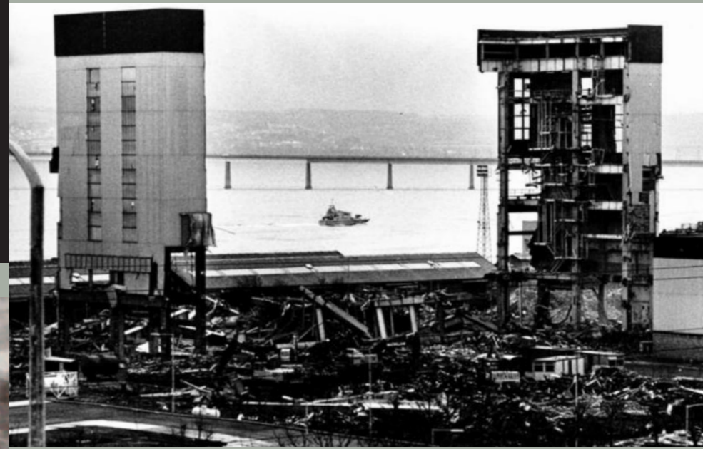
▲ Demolition of Carolina Port B
