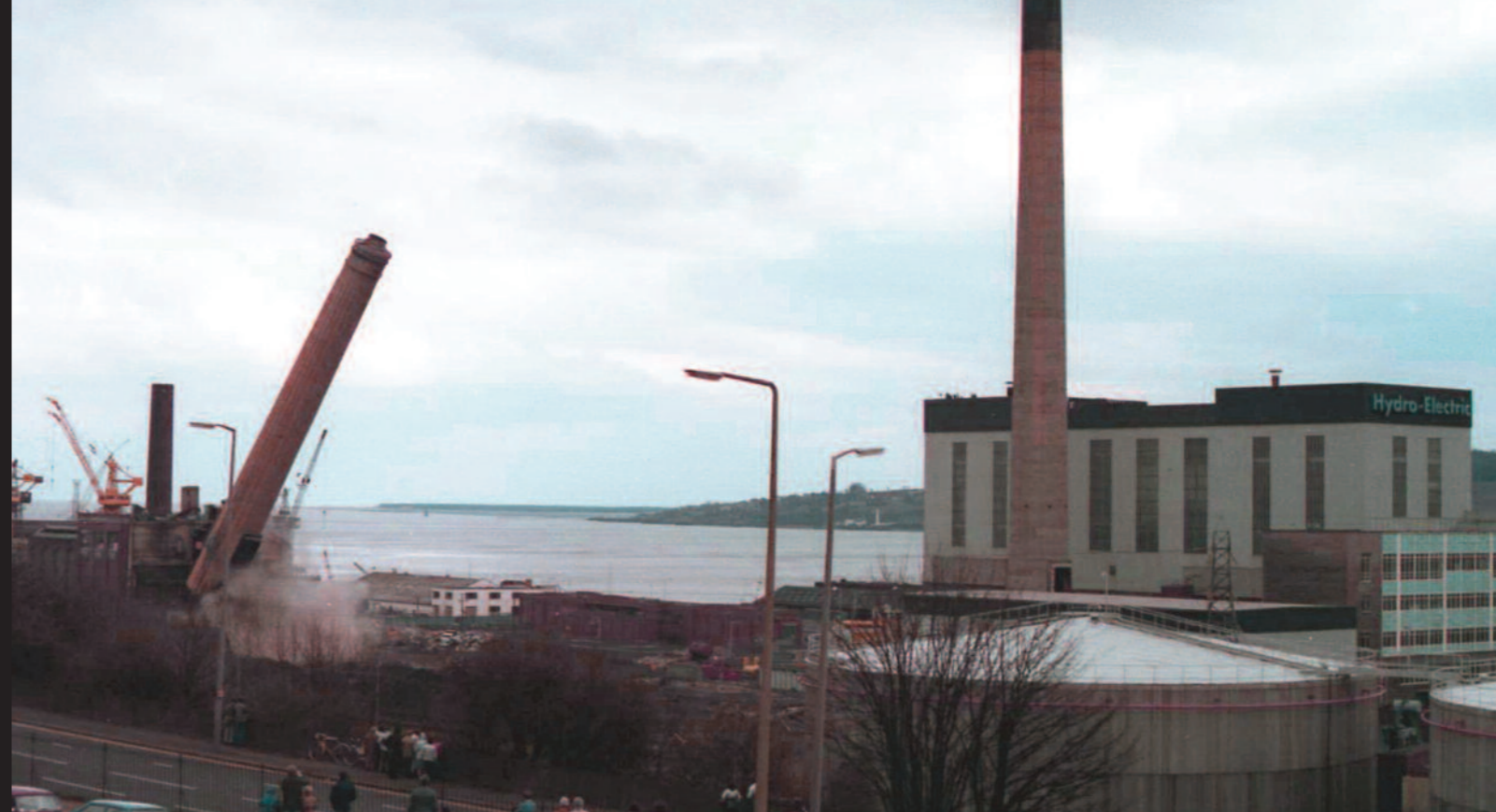
▲ Demolition of Carolina Port A
