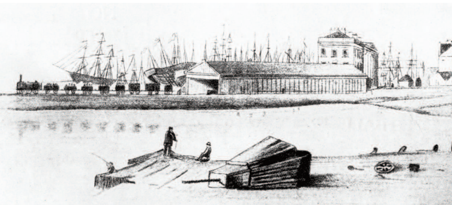
▲ This contemporary illustration is the only known picture of the Dundee and Arbroath Railway's Trades Lane terminus. It shows the station as it looked when opened in 1840, with a departing train heading out towards Broughty Ferry. In the background is the new Custom House and in the foreground is the old shoreline of the Tay, cut off by the railway causeway.
