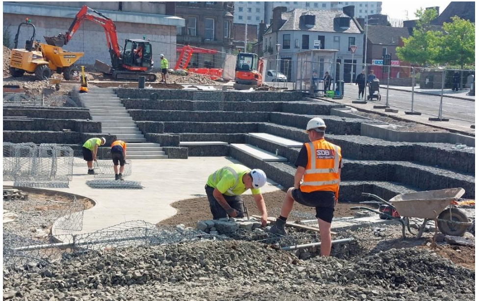
Lochee's new Aimer Square under construction. The gabion-packer is using his dyking hammer and a straight-edge to ensure a neat fit. Note the 'hearting' of crushed stone.
